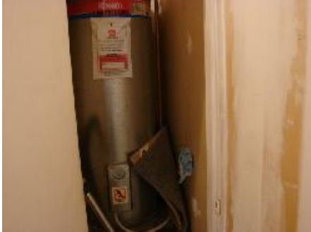
Hot water cylinder not restrained
