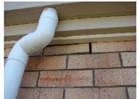
Loose brickwork
