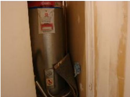
Hot water is not restrained
