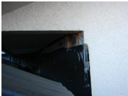
Flashing missing
