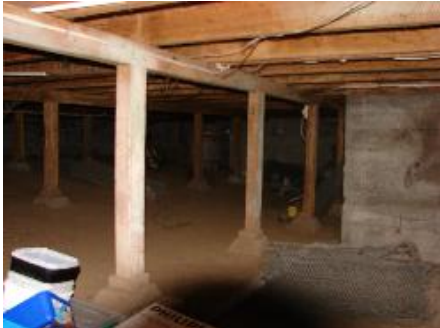
jack studs to bearers-no connectors
