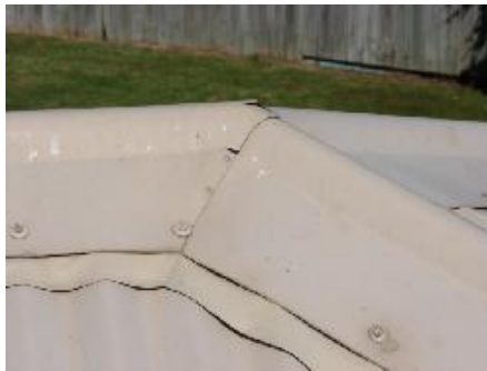
Ridge joints need sealant
