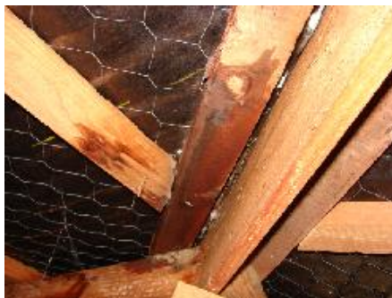
Roof Leak
