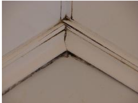
Plastic moulds around the bath that have broken and let the water through
