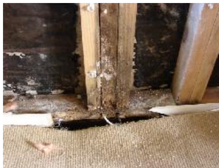
Leaking exterior wall
