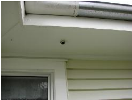
Replaced section of spouting
