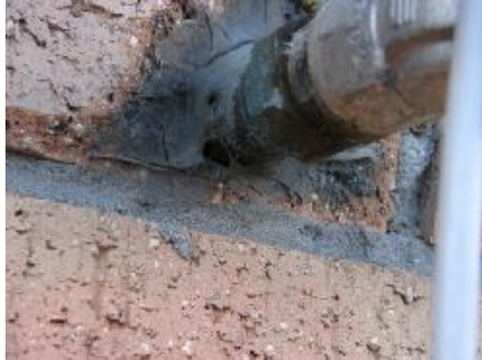
Poor sealing around pipework
